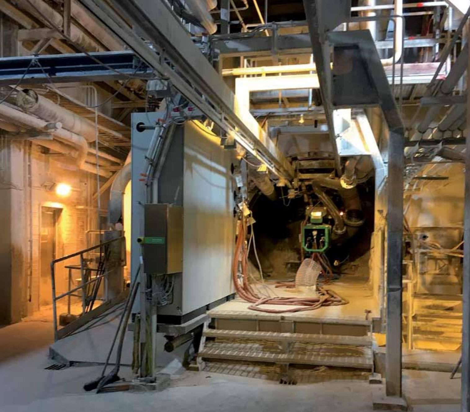
*Multi Fuel Lime Kiln Burner System for Metsä Board AB
